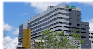
SILOAM HOSPITALS AMBON
